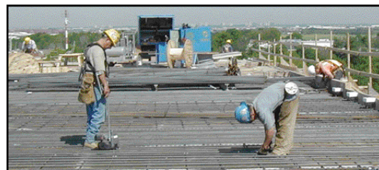
Tying rebar: Using a machine with an extension arm (left) or pliers (right).
