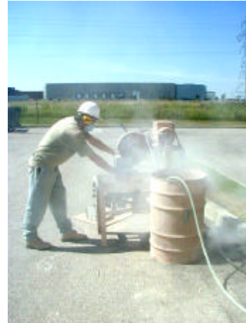
Figure 2: Much more dust produced by dry cutting
