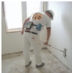
Figure 1. Sanding drywall with a pole sander.
