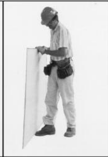
Lift sheet slightly and put toe under mid-point.
