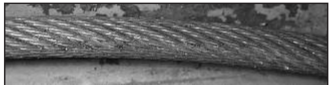
Outside of wire rope. It appears to be in good condition. See below.
